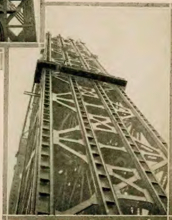
In the above photograph may be seen the steel skeleton of one of the towers. Each leg of the tower rests on a separate reinforced concrete base resting on bed rock and faced with granite. Arrows point to workmen.
