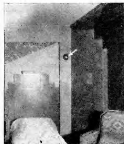
The arrow points to the outlet on the wall of the stateroom. The direction of the breeze may be changed by turning the nozzle.
