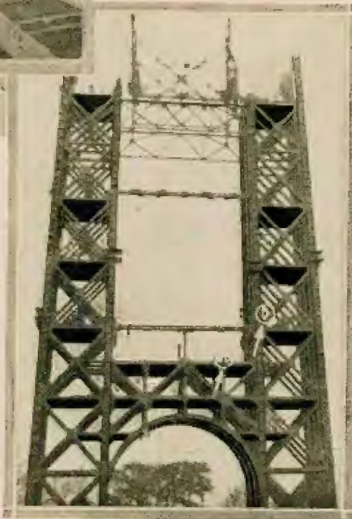
In the above photograph may be seen the steel skeleton of one of the towers. Each leg of the tower rests on a separate reinforced concrete base resting on bed rock and faced with granite. Arrows point to workmen.
