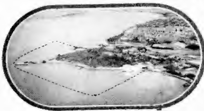
At North Beach, N. Y., the 55-foot hill was sprayed with a concentrated stream of water, which washed the earth into a sump hole, from which it was sucked and piped into the bay behind a bulkhead, to extend the airport area.
