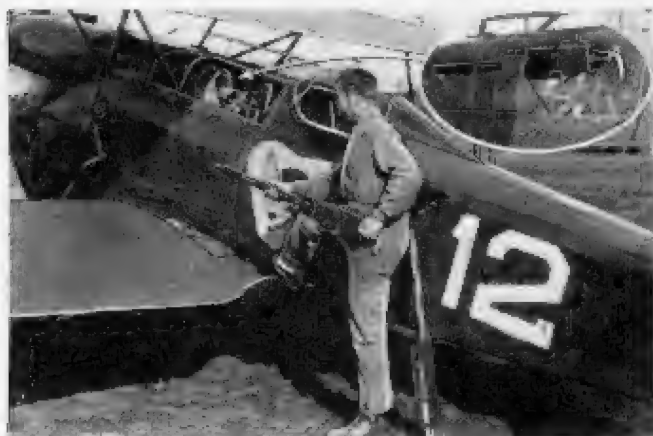
Installing a modern machine gun in the cockpit of an army pursuit plane. Inset—the gun in position.
